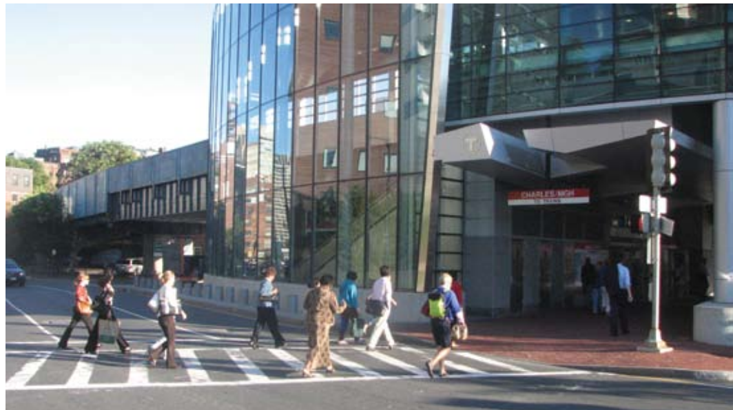
The newly remodeled Charles/MGH Red Line station was built to accommodate a connection to the extended Blue Line.
