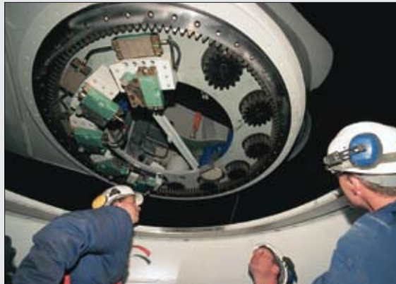
Workers inspecting a wind turbine.
