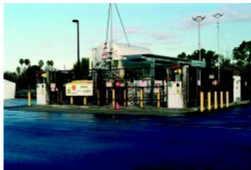
Hydrogen refueling station in Sacramento, California.
