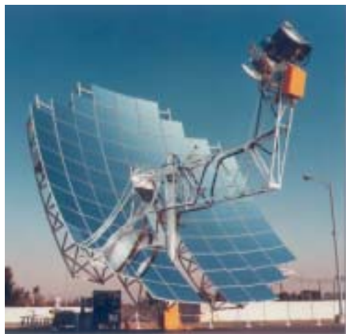
Stirling solar dishes efficiently transform solar heat into electricity.
