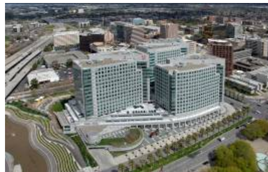
Software maker Adobe launched an aggressive effort to improve the energy efficiency of its San Jose headquarters, cutting per-employee electricity use by 35 percent. Credit: Proehl Studios® April 2006
