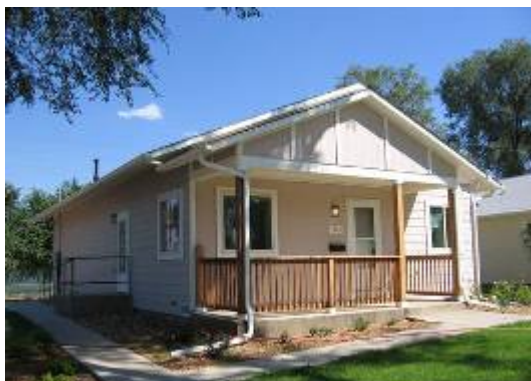
This Colorado home looks typical, but it holds a secret – it is a zero net energy home built by the Department of Energy for Habitat for Humanity. The home uses solar panels and a solar hot water system to produce as much energy as it consumes. Credit: DOE/NREL, Paul Norton
