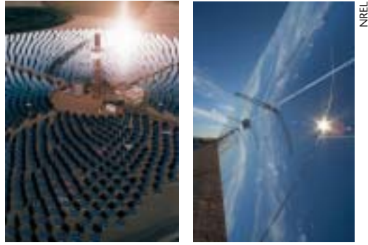
Solar Two (left), a power tower in the desert southwest, demonstrated the feasibility of storing heat from the sun to generate electricity at night. For over 10 years, parabolic solar trough power plants (right) have produced electricity for California.
