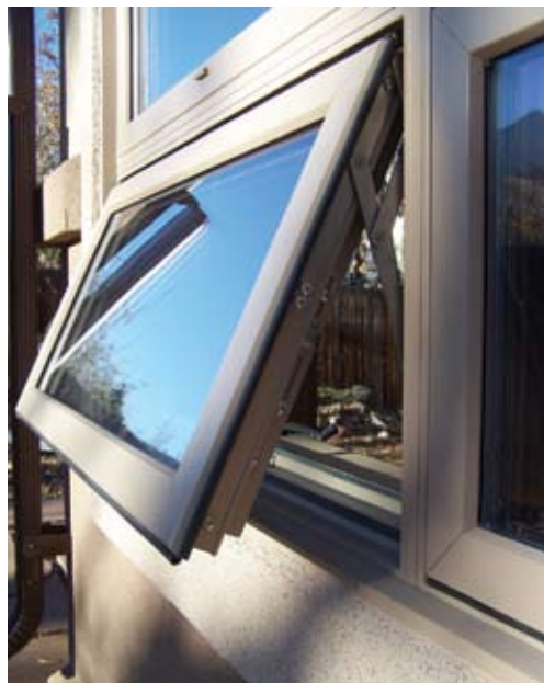
The Graham home in South Boulder uses highly efficient technologies, such as this “heat mirror” window, to practically eliminate winter heating costs. (Credit: Ecofutures Building, Inc.)
